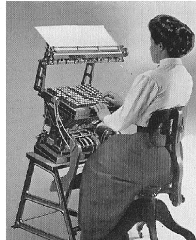
Automatic Punching Machine – Census Model 1910
